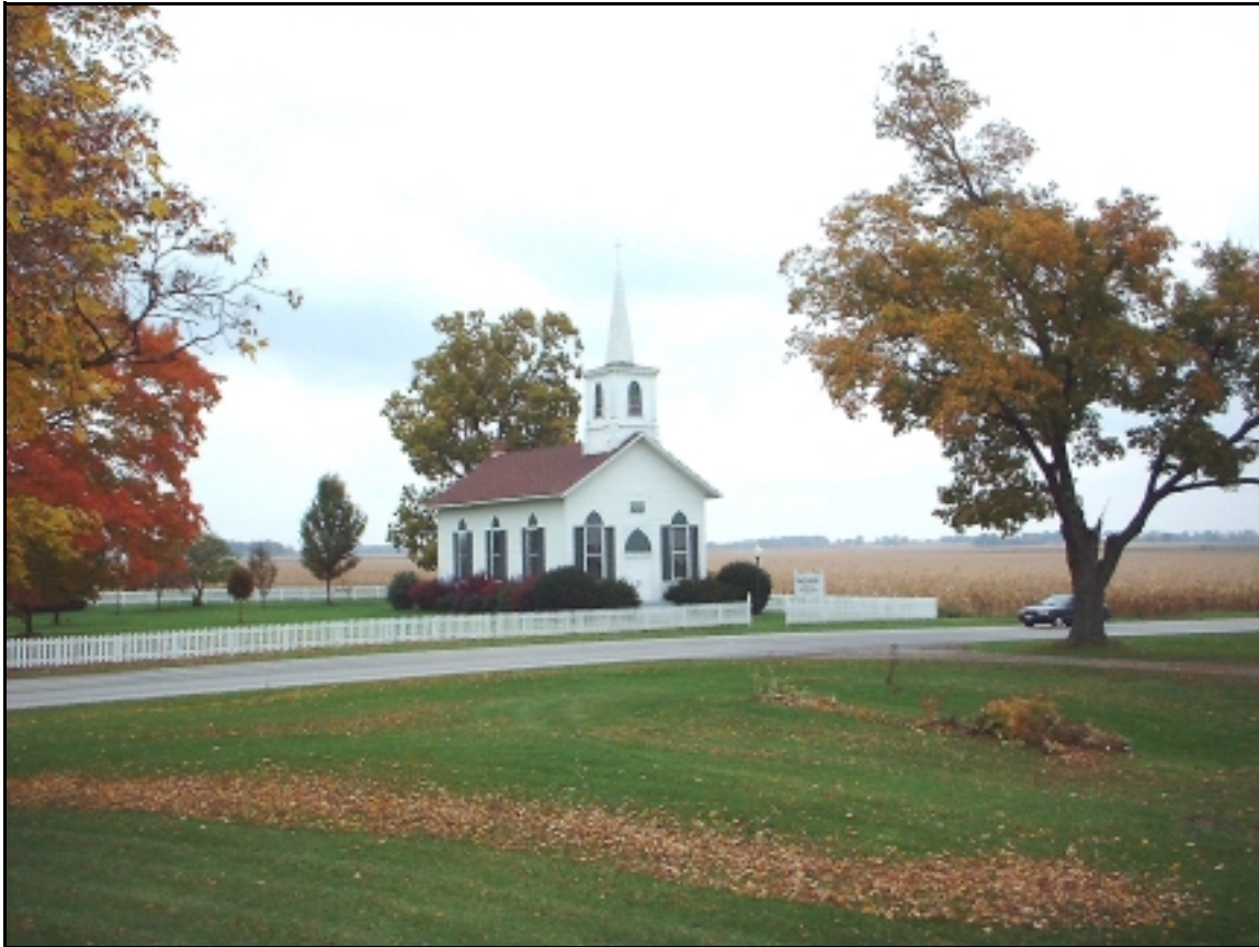
Hunt’s Corners Church, October 2002. View shows the newly repaired picket fence. Photo courtesy of Kurt Heyman.
